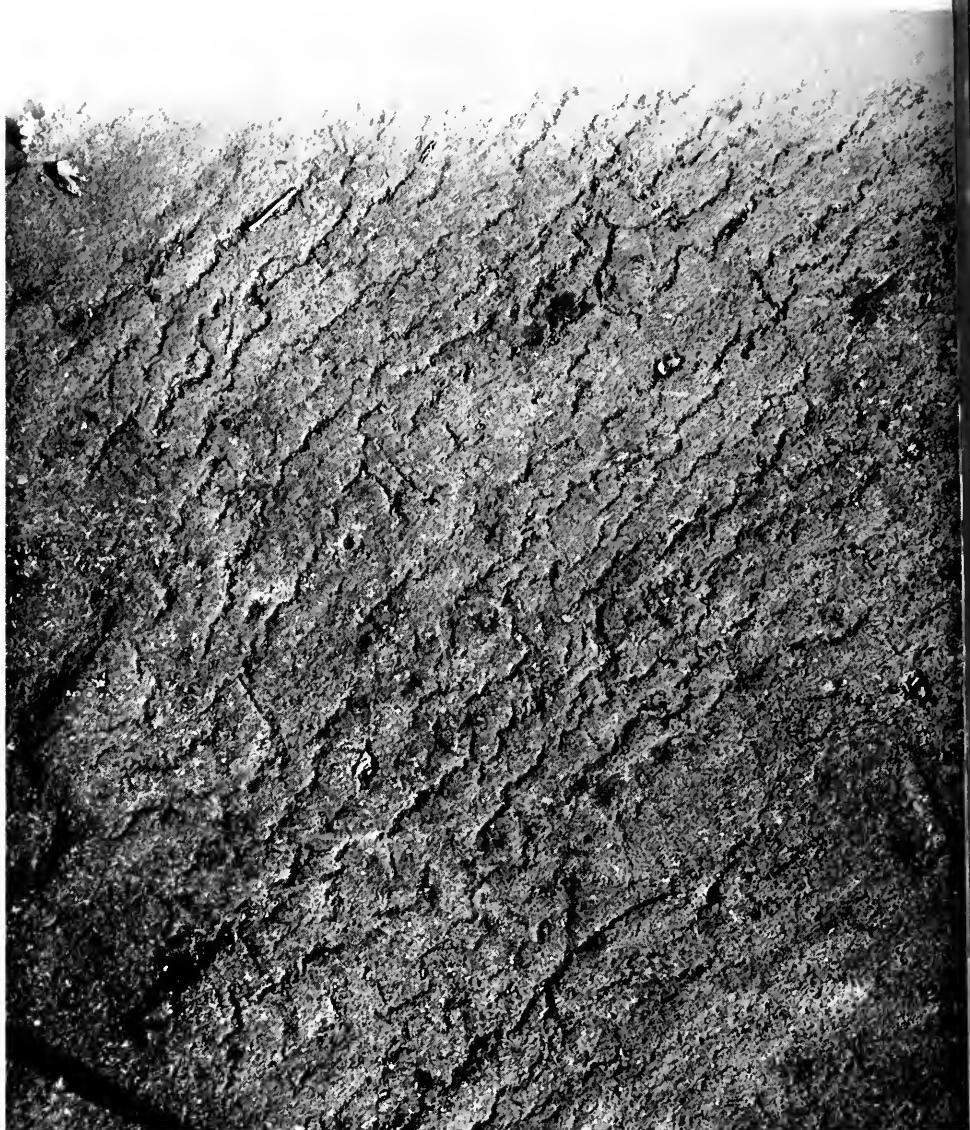
Linden Ave., showing deeply "wrinkled" typical surface. August 10, 1909.
